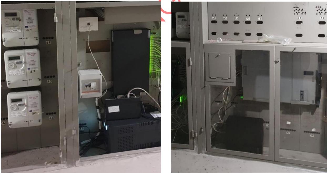
Figure 86: The physical connection detail of the smart meters to the computer.
