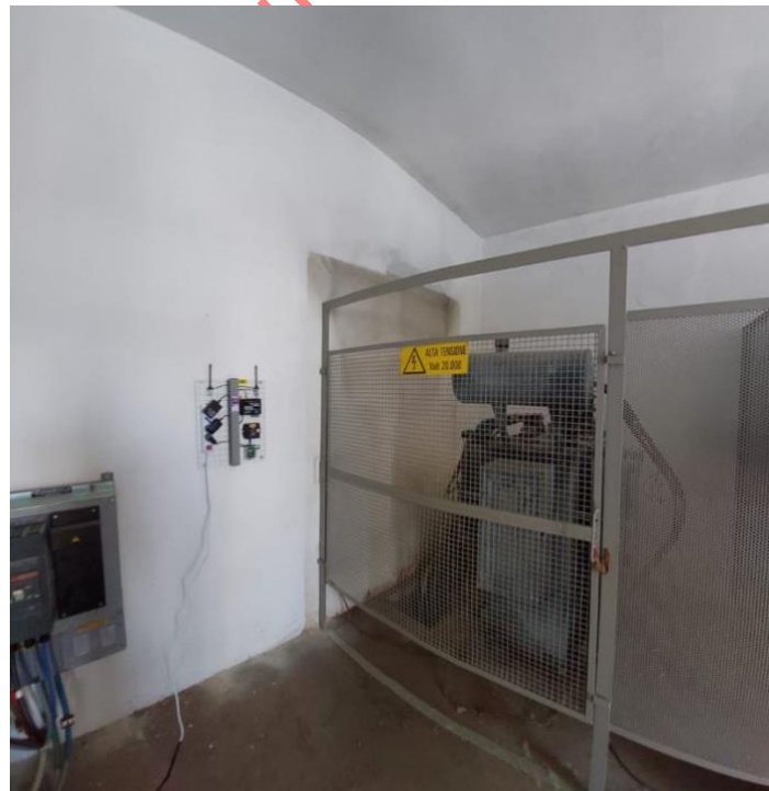
Figure 1: Transformer and a part of the secondary cabin.
